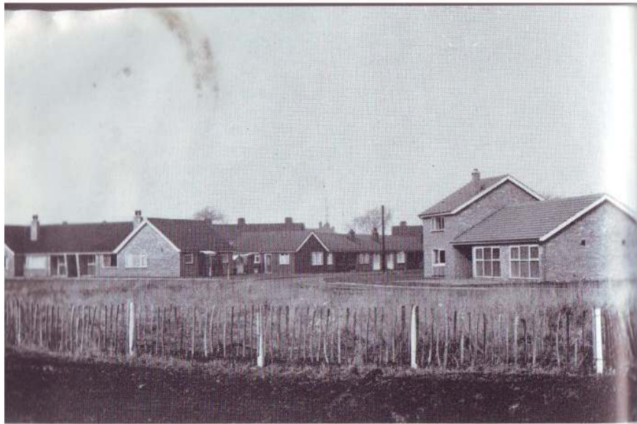
O.P. Homes and Community Centre, Snaith Photo: Norman Burnitt
