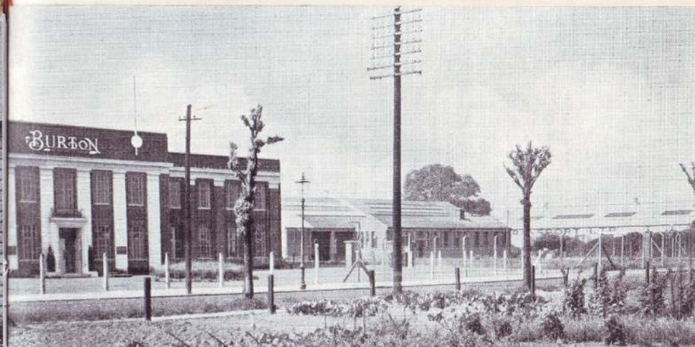
Part of Rawcliffe, Road Industrial Estate
