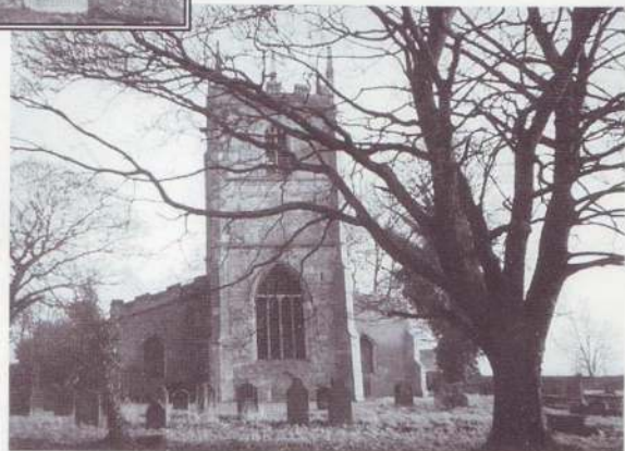
Right: St. Mary's, Whitgift. Notice the door in the tower; now only half of it is above the ground due to settlement over the centuries. Inset (above): three minutes past 13 o'clock!
