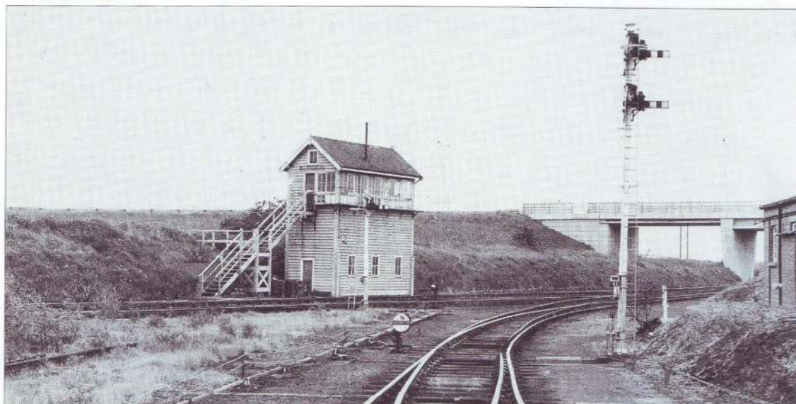
Moving down into the yard, we turn round to look westwards. The date is 7 June 1986. The road bridge in the distance was the vantage point for our earlier photographs. The splendid signal box is Goole Goods Junction box which opened in 1891 as a replacement for Goole Goods Yard box. Its original 40-lever L&Y frame was replaced in November 1958 by a 55-lever McKenzie & Holland frame; the box was downgraded to a points box (non-block post) in July 1978 and closed completely on 20 March 1989. It was later demolished. Note the single-arm shunting signal near the 'box, the two-arm shunting signal on the right, and the mess cabin for the shunting staff on the extreme right. Virtually concealed behind the signal box are two elevated sidings, though the embankment on which they run is discernible.
