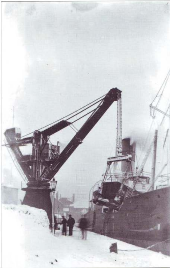
A 50-ton hydraulic crane was installed in Stanhope Dock in 1892 to be used for heavy lifts and coaling ships by lifting railway wagons from adjacent tracks. This photograph by E. Thompson, shows the crane in action in the 1910s. Another photograph of the crane in use appeared in Archive No 9. BM
