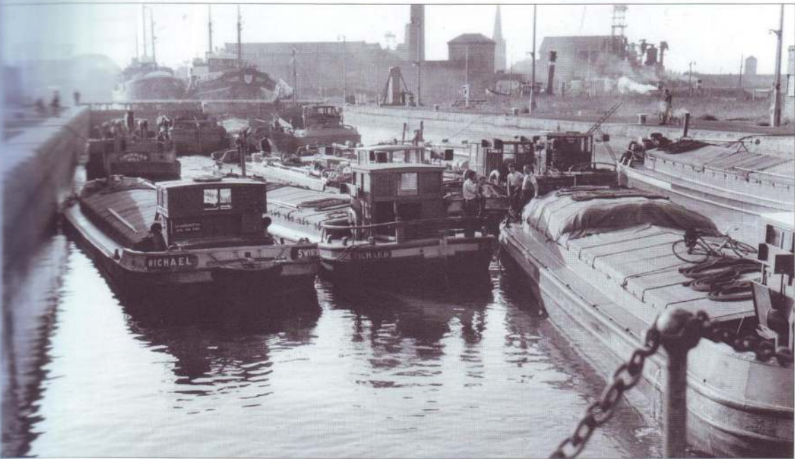
Inland waterway craft used one of the locks to pass between river and canal. This photograph, taken in the 1950s shows craft in double figure numbers penning up the 360ft x 80ft Ocean Lock prior to heading into the docks or passing through to reach the A&CN. Michael is loaded with wheat for Rotherham, collected from the silo in Hull's King George Dock. One of Everards' ships and one of Hull Gates' are waiting to lock out into the river. NT
