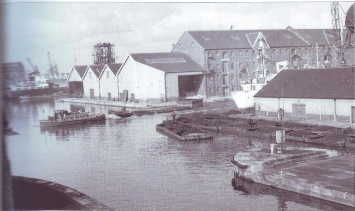
Compartment boats are here being moved about the docks by one of the diesel tugs in March 1965, close to Aldam Dock's No. 3 compartment boat hoist. Notice the 'jebus' placed immediately behind the tug to lift the first few pans and deflect the tug's wash beneath them. This was customary in front of the tug when empty pans were being taken to the collieries to be loaded. To the right, loaded puddings wait to be tipped at the hoist. Norman Burnitt
