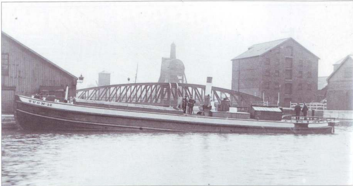
The general merchandise tows were hauled by either cargo-carrying tug/barges (as in the previous illustration) or 'Merchandise' tugs. Tug No. 12 , one of the former vessels, built by T. Scott & Company at Goole in 1891, is shown here in the 1900s posed against Lowther Bridge in the docks with a hydraulic accumulator and compartment hoist No. 2 in the background and the East Salt shed to the right. WMG
