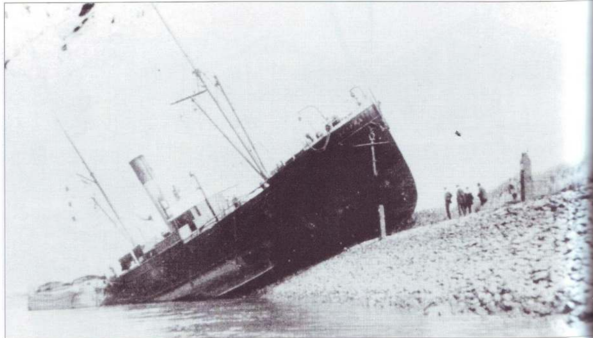
The Goole Steam Shipping Company's s.s. Altona is shown aground on the lower Ouse training walls in August 1908. The walls were constructed by the A&CNC to deepen the channel using blast furnace slag brought from Teesside in hopper barges. Giant pitch pine piles 40ft long were driven into the river bed at intervals and the slag tipped around them. Construction began in the 1880s and, by 1894, 2,000-ton capacity ships could reach Goole, whereas previously 700-ton cargoes were the maximum. The work was finally completed in 1935. BMG
