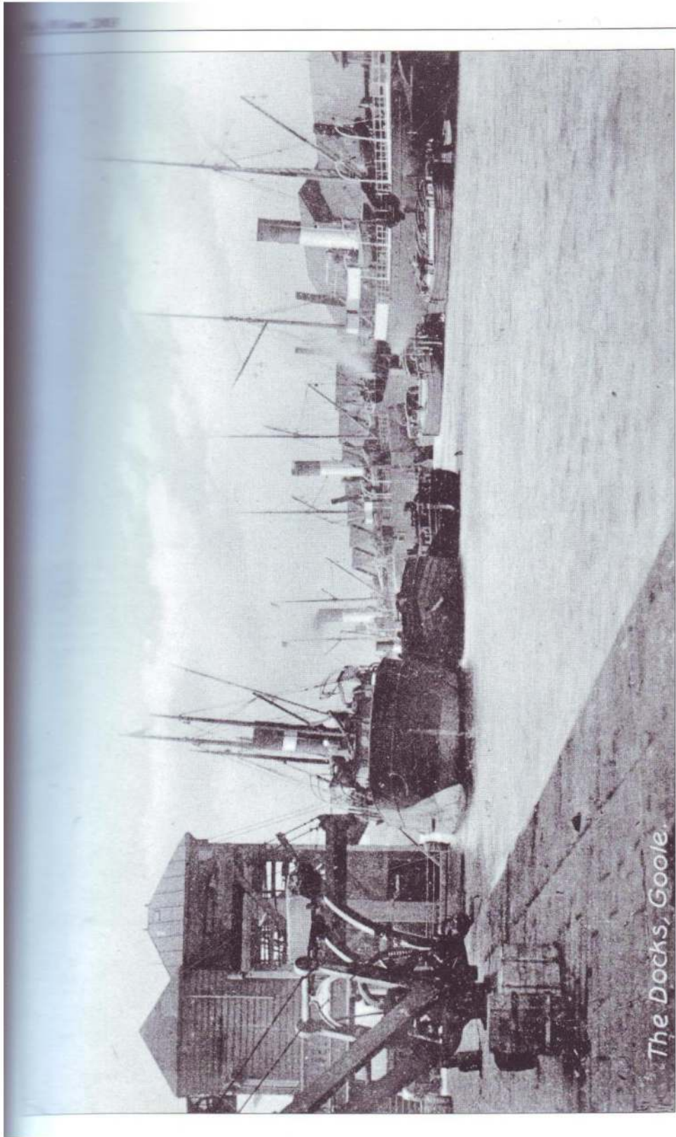
The Lancashire & Yorkshire Railway came onto the docks in 1848 with the opening of Railway Dock and was followed by the North Eastern Railway in 1869. Coal was the major cargo brought by rail and cranes and wagon hoists to complement the compartment hoists were built to transfer it to the holds of ships. The 1879-built wooden-roofed Ormerod Grierson Hoist is shown to the left of this 1900s view looking north along Railway Dock and into Slanhope Dock. Three of Gooles Steam Shipping Company's vessels may be seen being worked on the other side of the dock.
