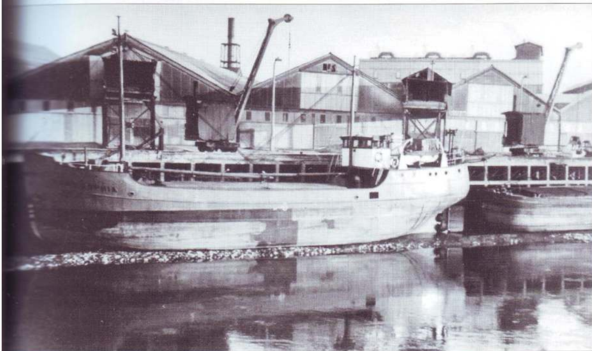
The berths at Fisons' Wharf on the south bank of the fast flowing tidal Dutch River tended to dry out at low water as shown on this picture when the Lady Sophia . Shipping bound for the wharf from the Ouse usually approached it stern-first, just before high water, for best control. Even so, there have been several accidents at the swing bridge below the wharf with craft jamming it open, to the great inconvenience of residents of Old Goole. BM
