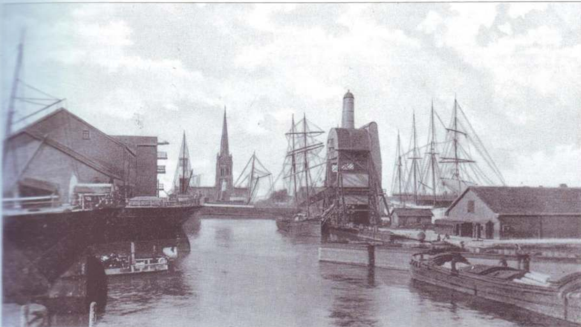
Looking north, this postcard view shows No. 3 compartment boat hoist that was installed during 1900 in Aldam Dock, with St John's church visible as it is on so many dock views. At busy times, the hoists often worked until midnight. This hoist acted as reserve to No. 5 in South Dock for the final few years before the Pudding traffic ended in the mid-1980s. MT
